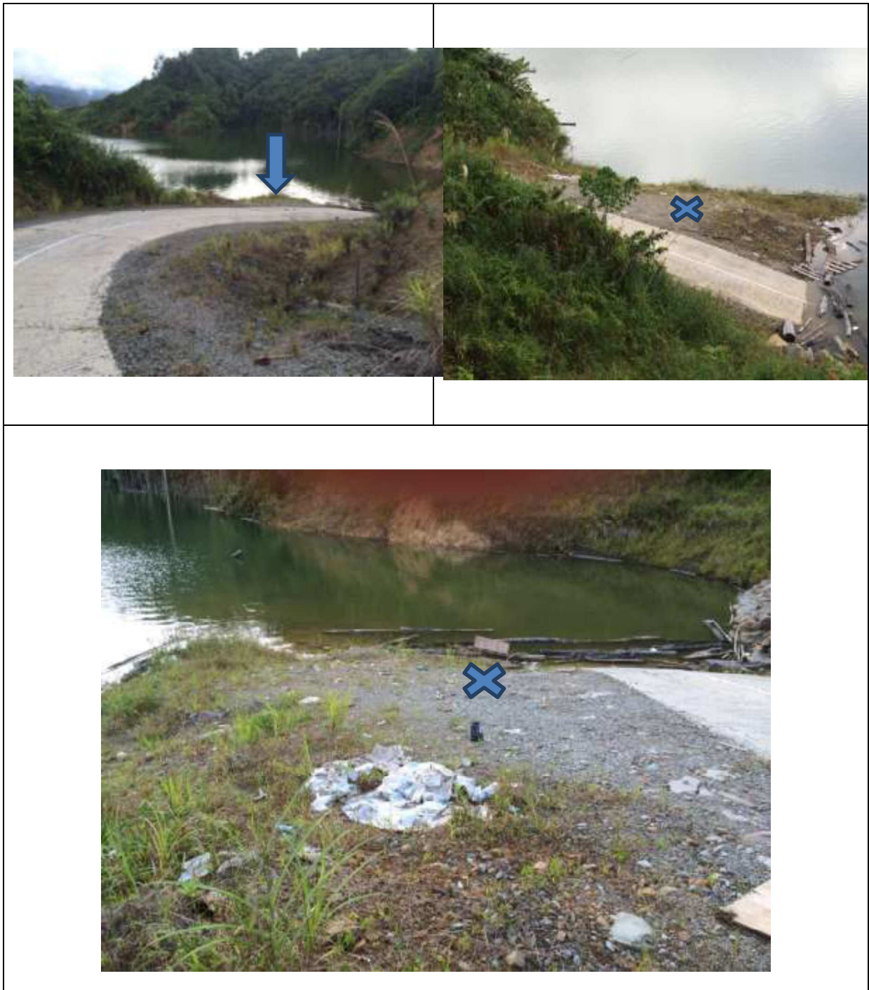
Combination of the above picture shows the location of the floating platform and all of its related structure as mention in the scope of work. Actual to be confirmed on site.
